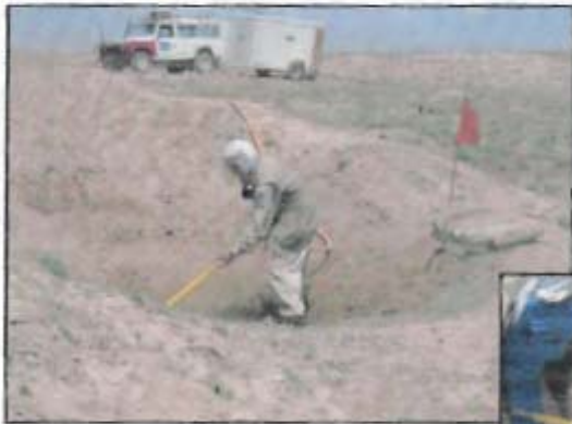
Airspade operator excavating ammunition pit.
