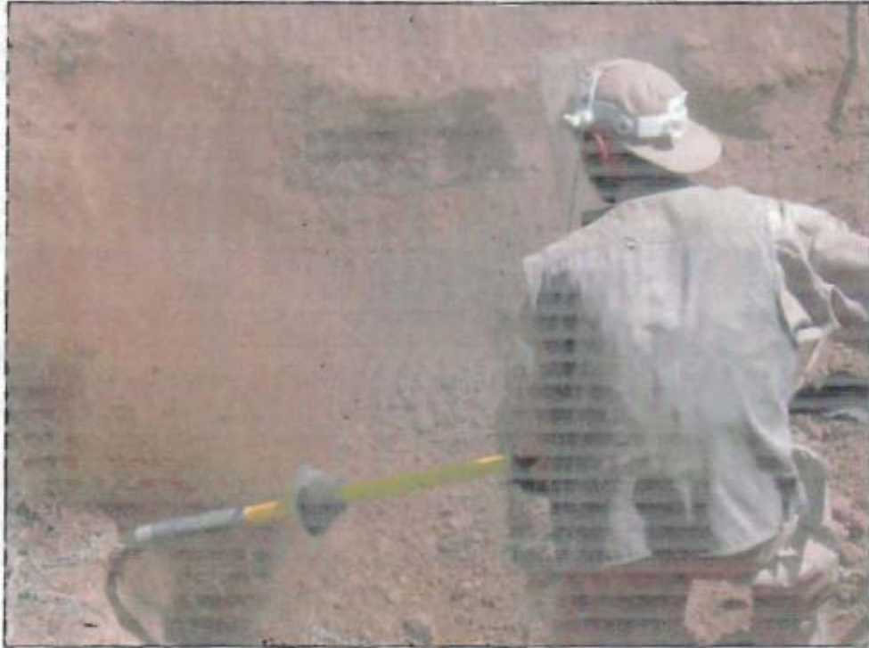
Airspade operator excavating ammunition pit.
