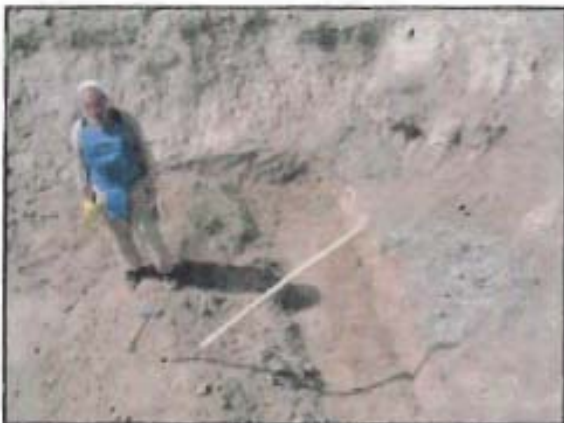
Manual excavation site, deminer uses trowel and shovel for the removal of soil to uncover munitions.
