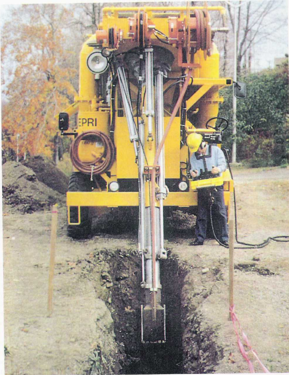
Soft Trencher — A 1994 advancement in vacuum excavating technology.
